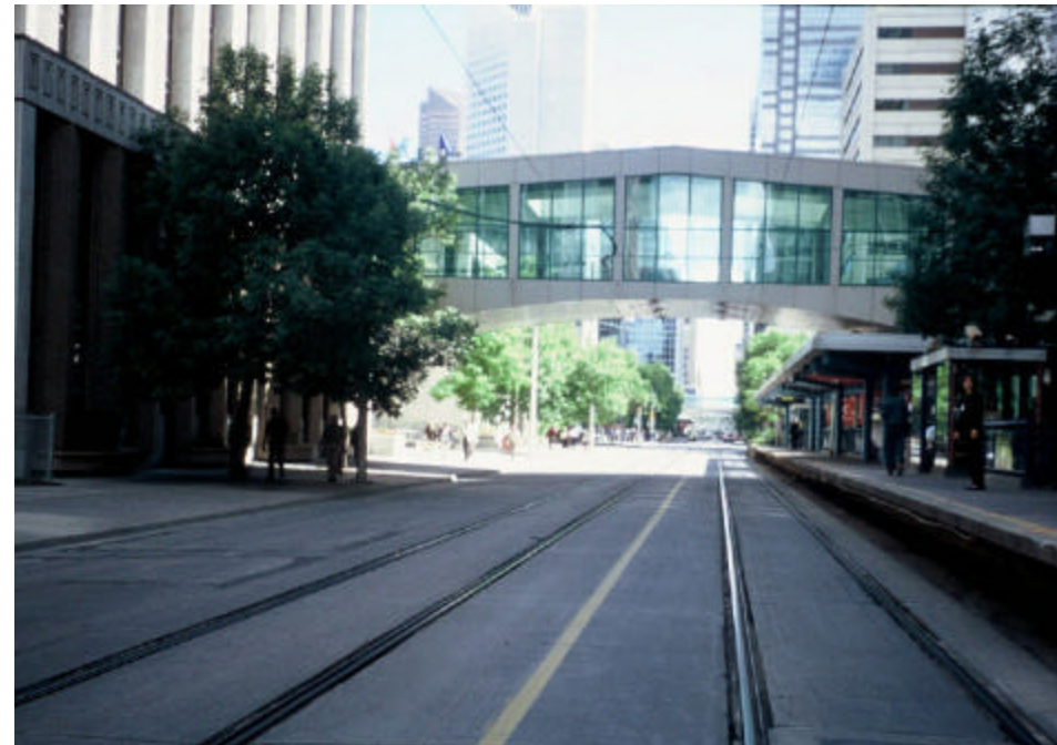
Figure 2a, looking west near the 6th Street W Station (Block F).
