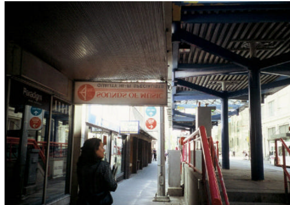
Figure 2e, existing sidewalk at 2nd Street W Station (Block J)
