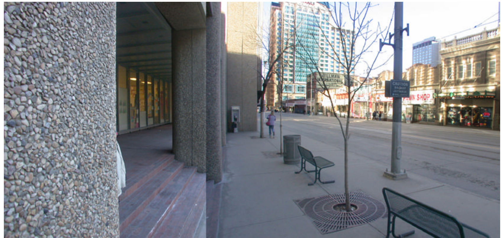
Figure 36, Existing Raised Arcade and Storefronts at the Len Wery Building
