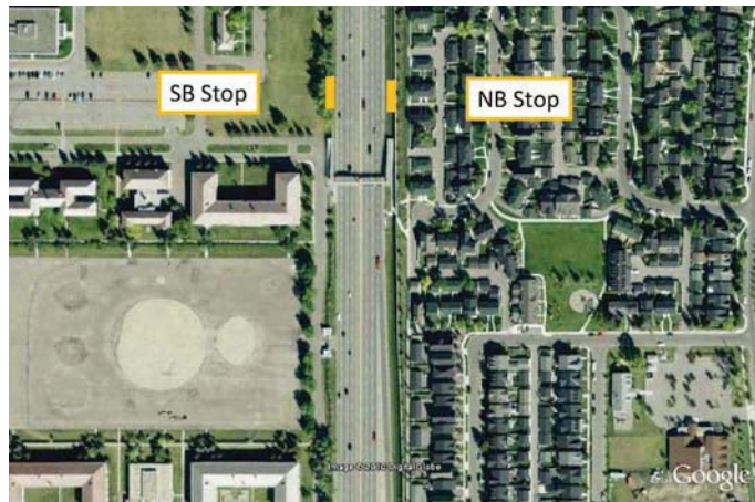
Figure 5: Crowchild Trail at Dieppe Avenue Pedestrian Overpass
